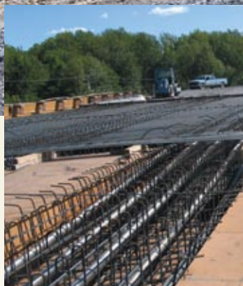
Structural work continued throughout the winter and is therefore quite advanced.
