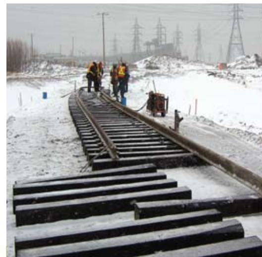
Installation of ties under the rails by the Transports Québec contractor
